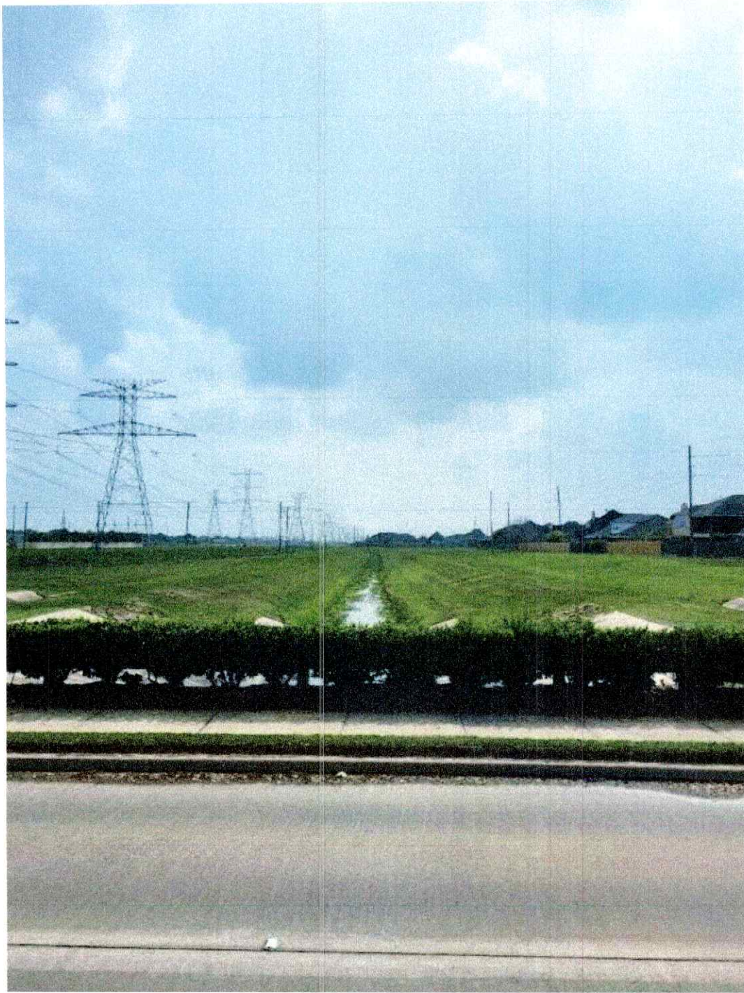
Channel B: Work Completed: 3-11-24
