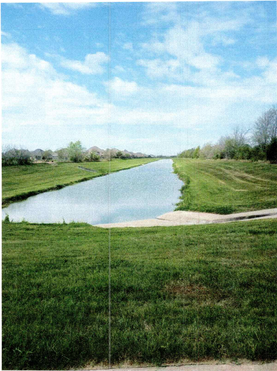
Lake 10: Work Completed 3-11-24
