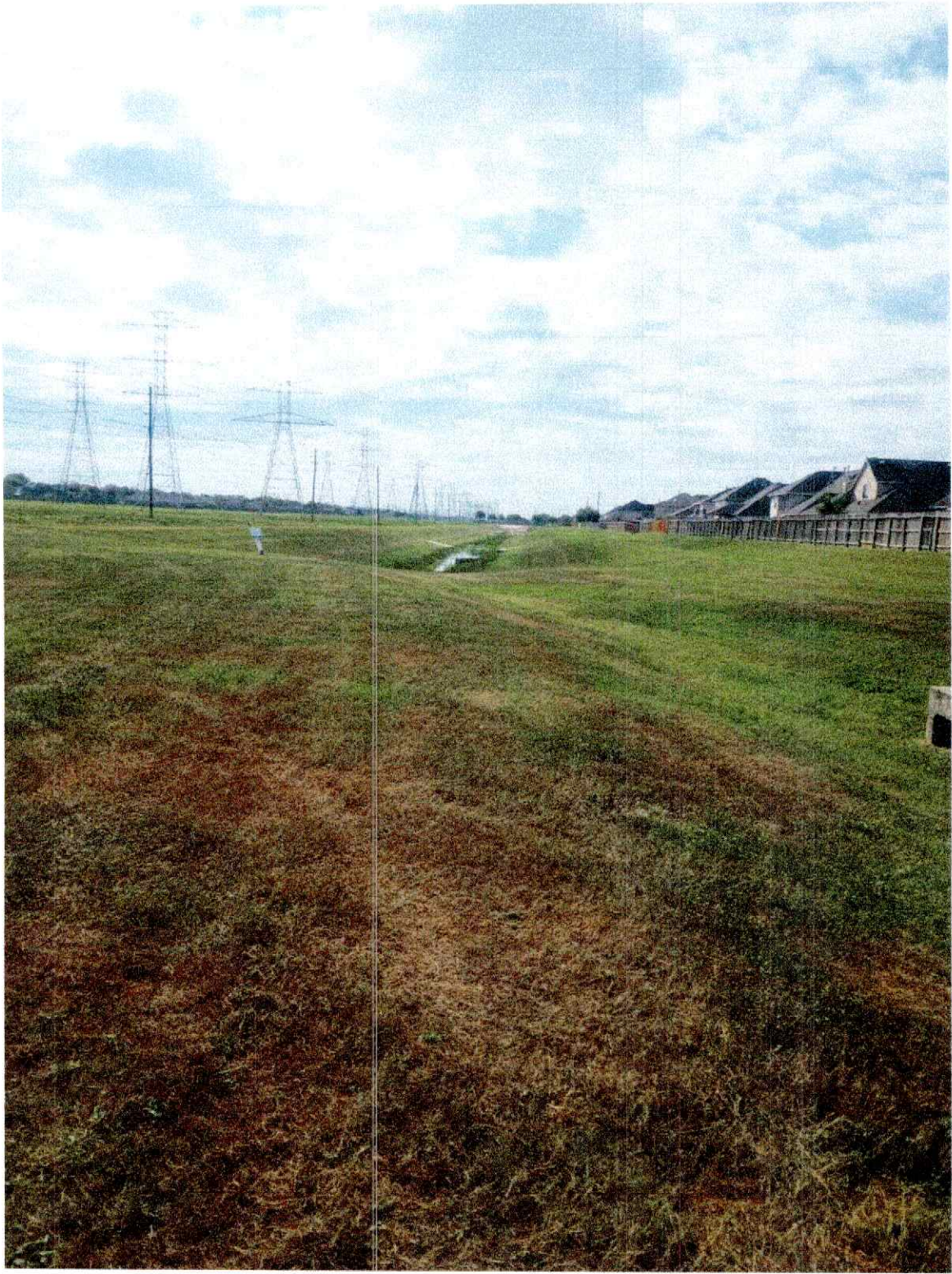
Channel D: Work Completed 3-8-24
