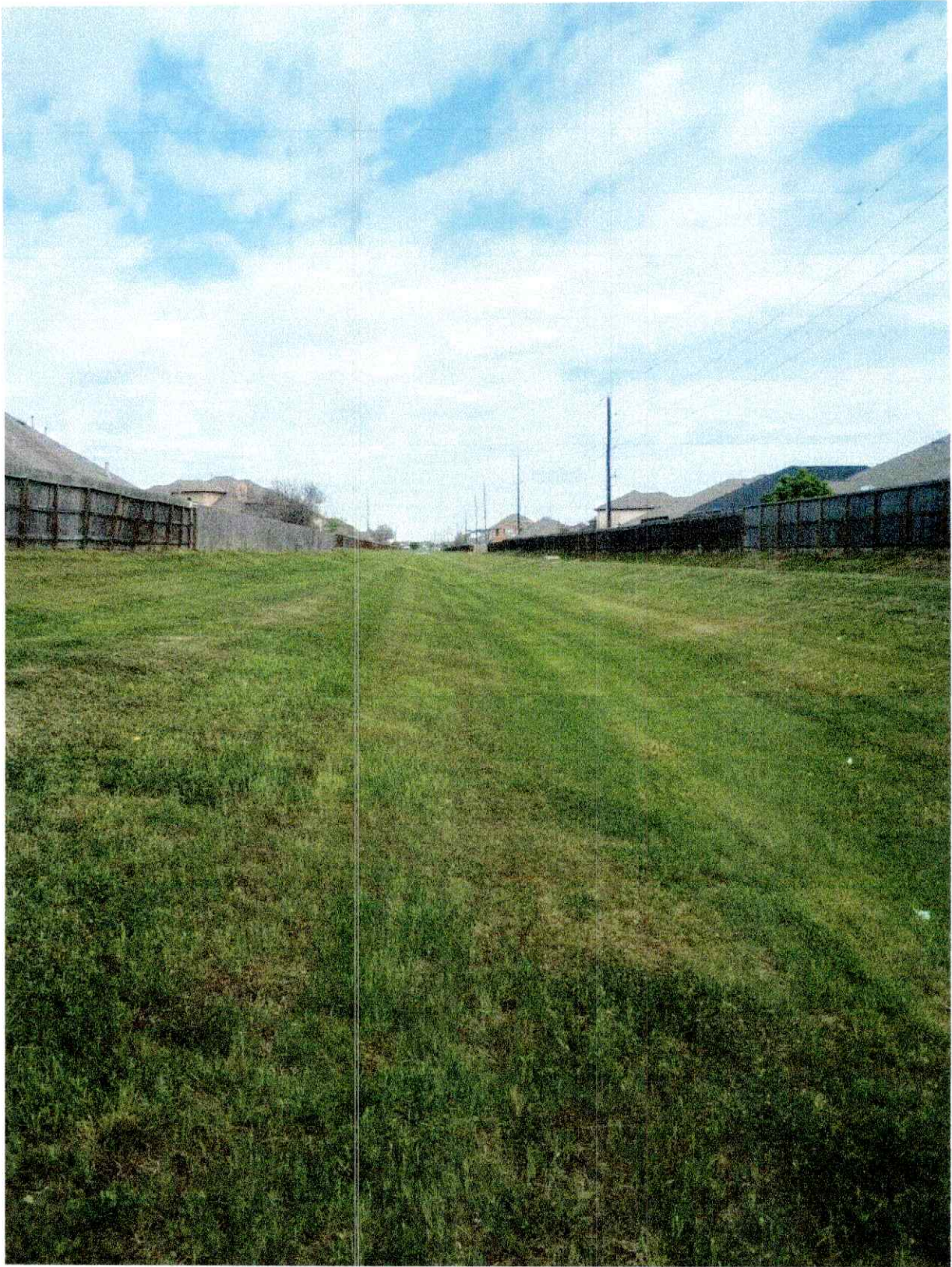
Lake 10 Channel: Work Completed 3-11-24
