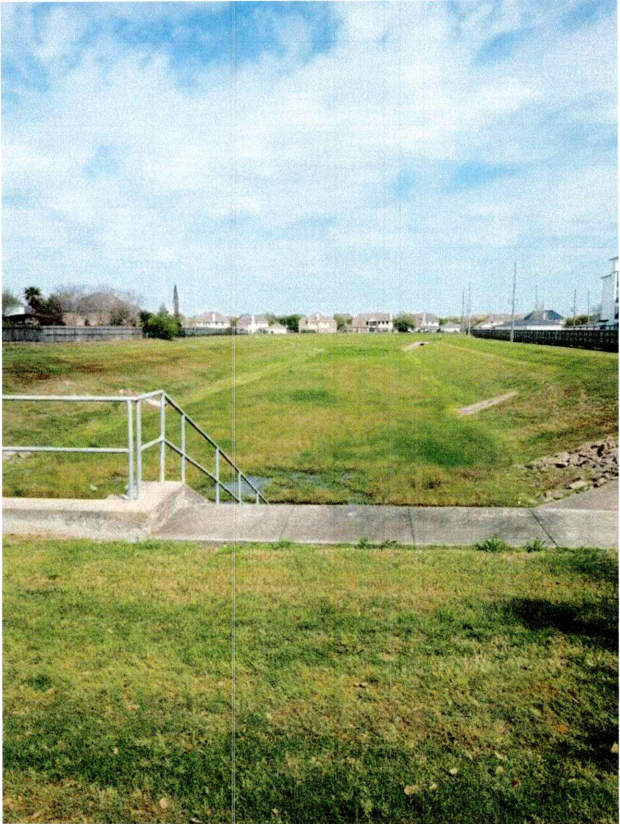
Channel A Outfall: Work Completed 3-11-24
