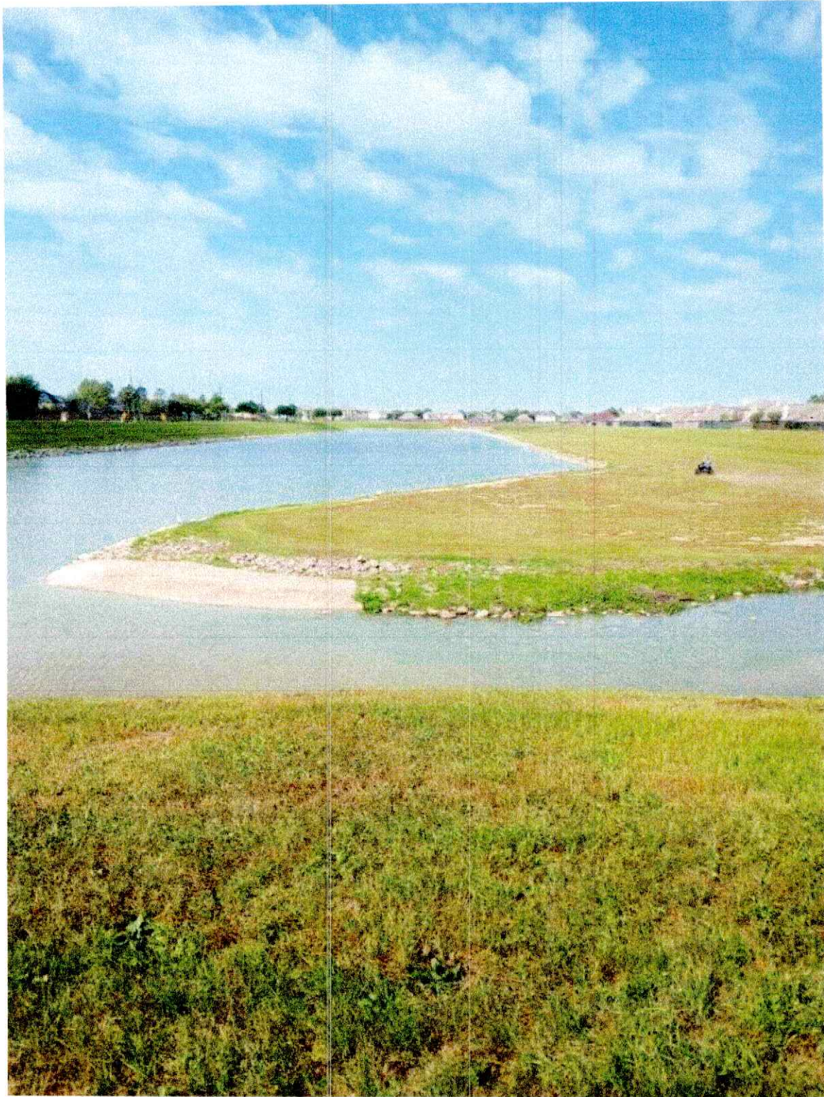
Channel C: Work Completed 3-8-24
