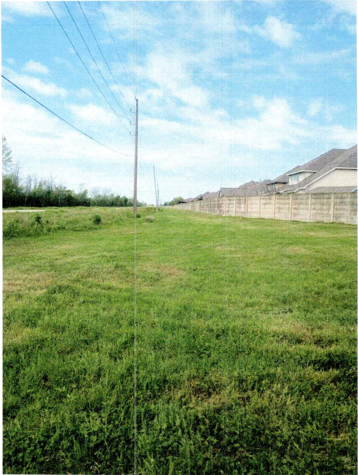
Lake 10 Fence Line: Work Completed 3-11-24
